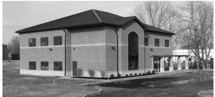
WCC's new Regional Services Center in Hebron, Kentucky
